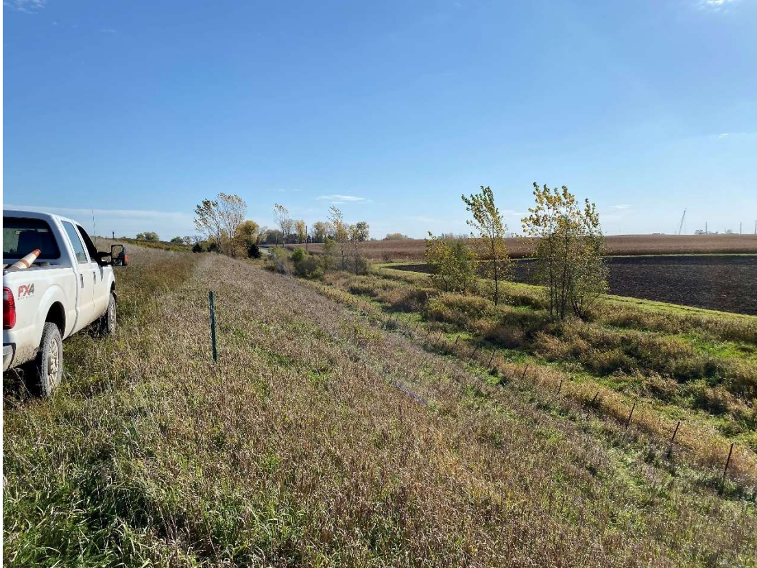
Location 7 – Looking East, Phase 2 Southern Berm
