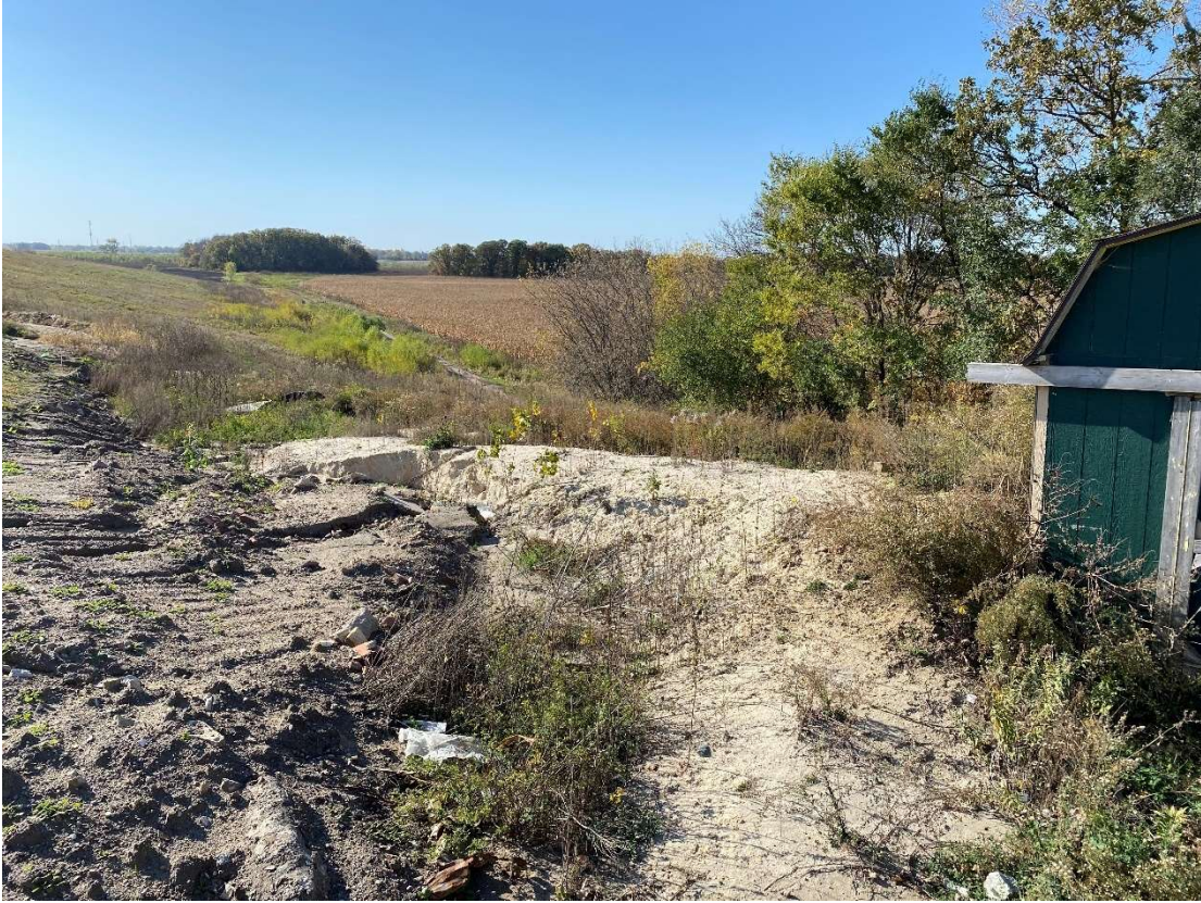
Location 1 – Looking Southwest, Phase 4 Anchor Trench
