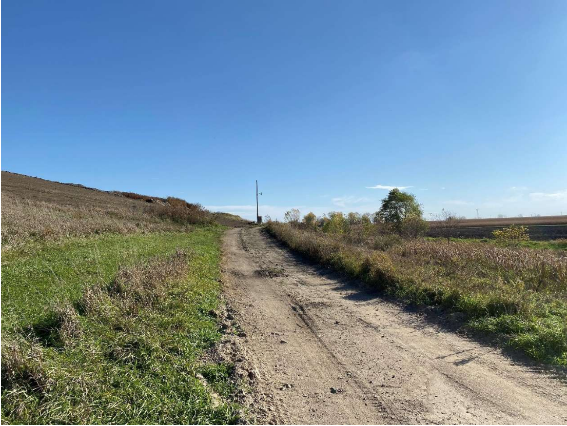
Location 5 – Looking East, Toe of Phase 1 Southern Slope
