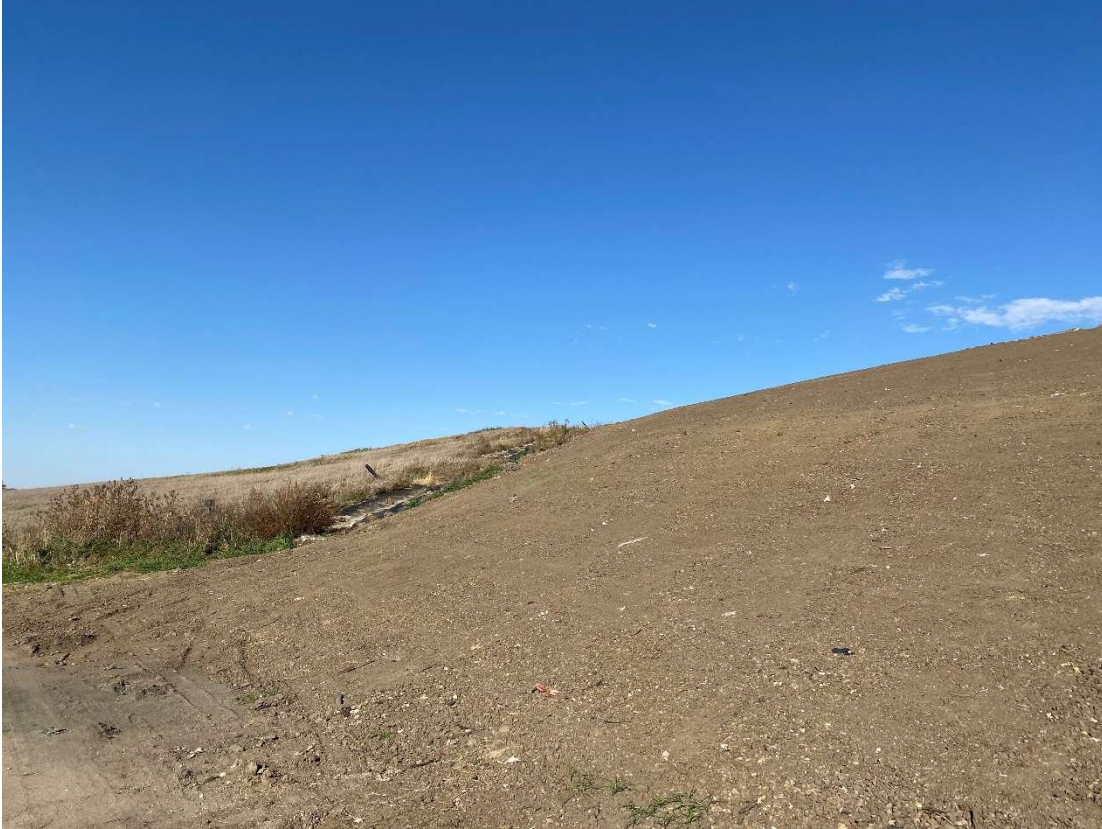
Location 6 – Looking West, Phase 1/2 Overlay Liner & Southern Slope
