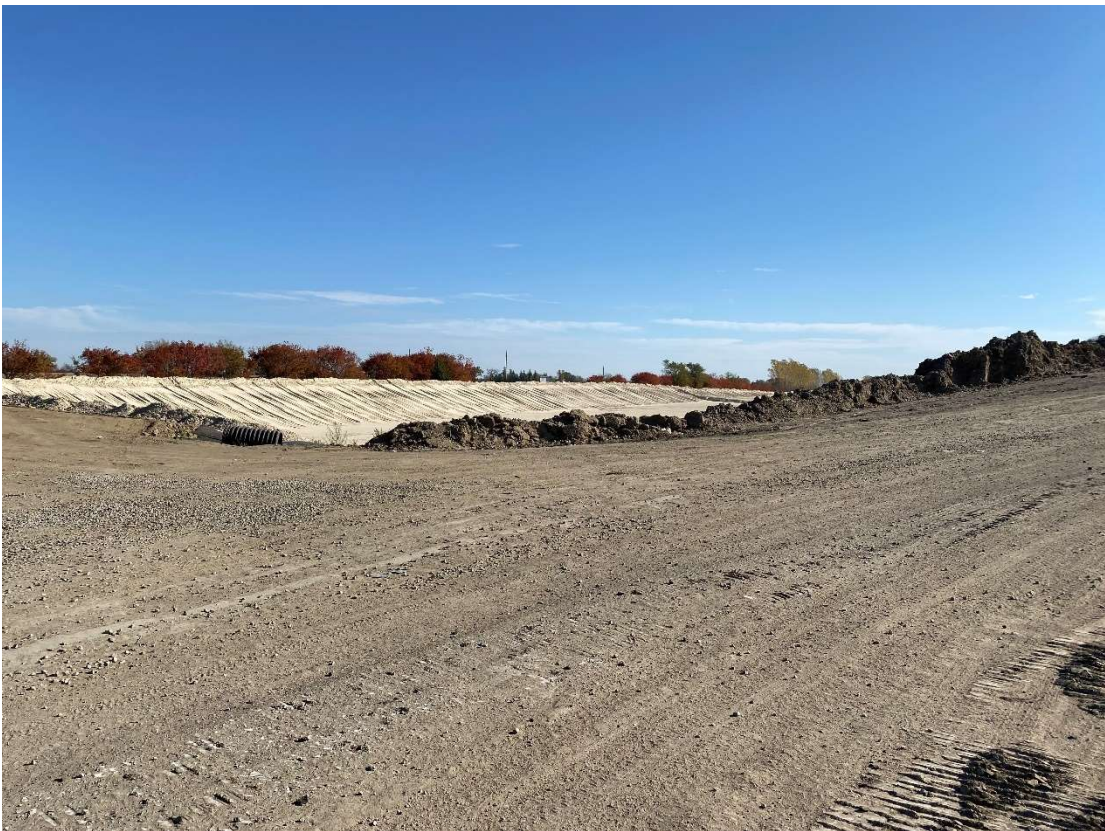
Location 2 – Looking Northeast, Phase 4 Anchor Trench
