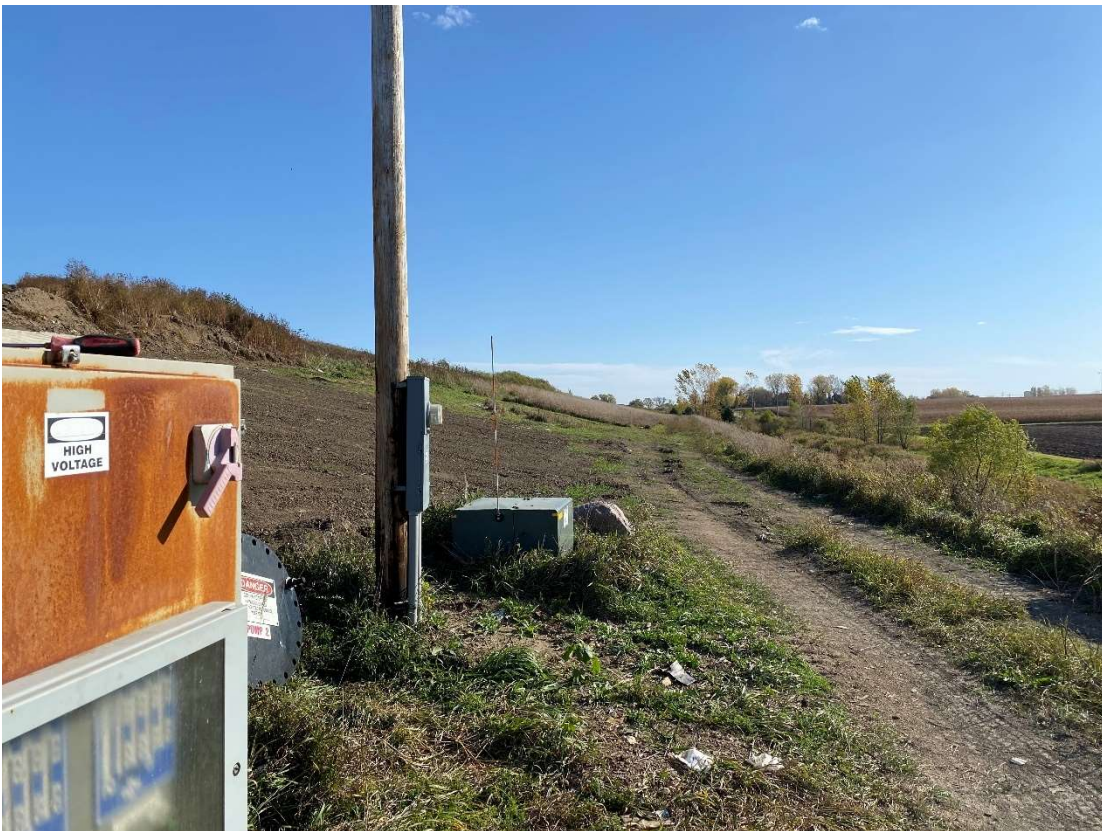
Location 6 – Looking East, Phase 2 Southern Slope
