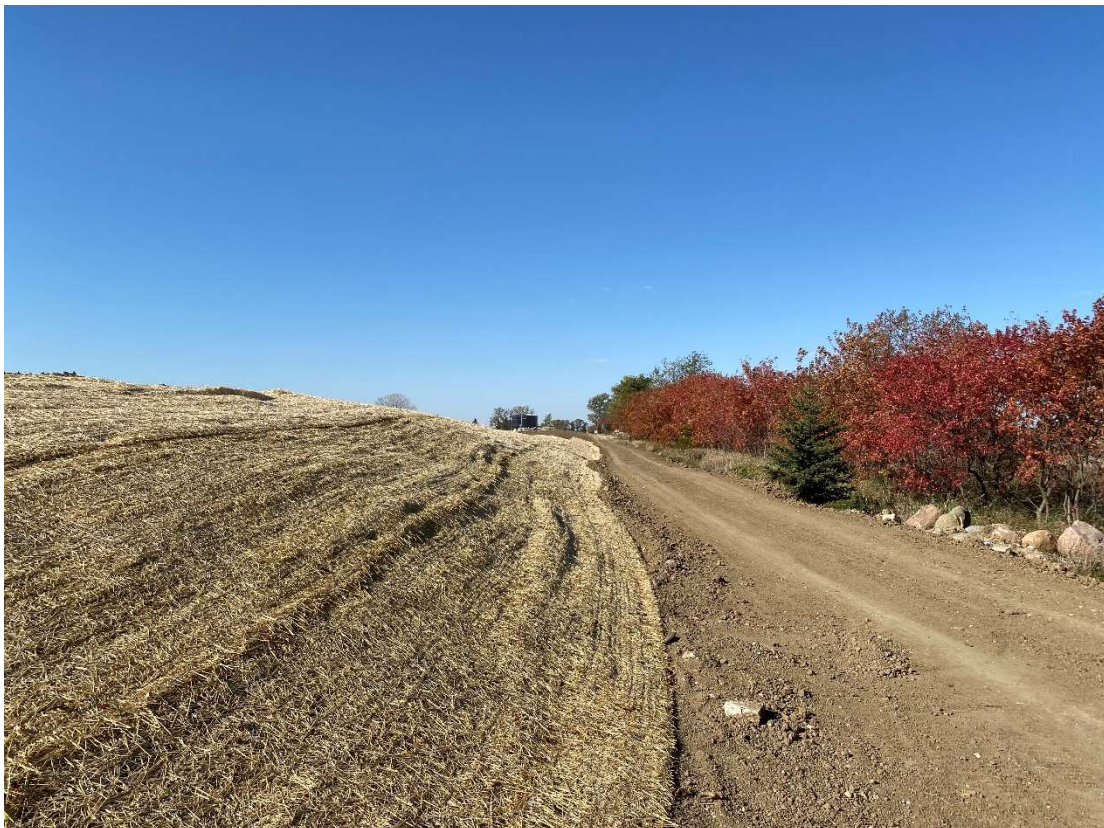
Location 13 – Looking West, Phase 5 Toe of Berm
