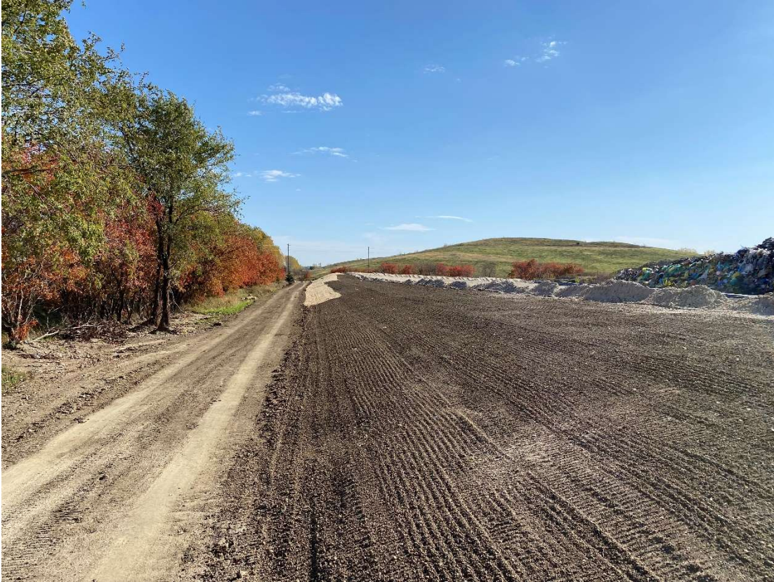
Location 14 – Looking East, Phase 5 Toe of Berm
