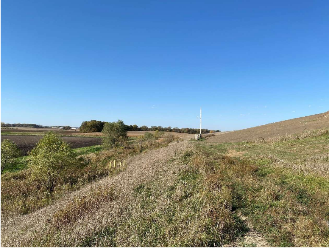
Location 7 – Looking West, Phase 2 Southern Berm
