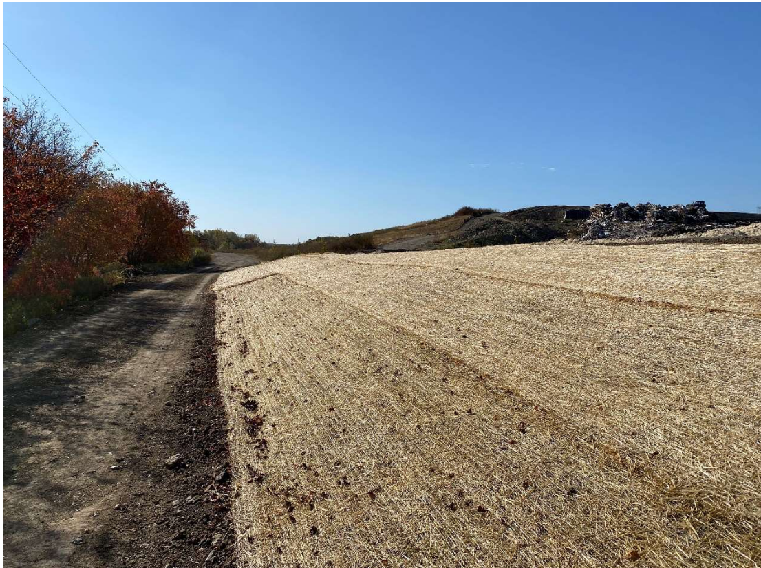
Location 13 – Looking South, Phase 5 Toe of Berm
