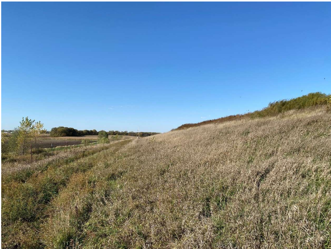
Location 8 – Looking West, Phase 2 Southern Perimeter Road and Slope
