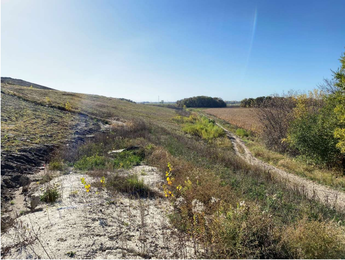
Location 2 – Looking South, Phase 3/1 Western Perimeter
