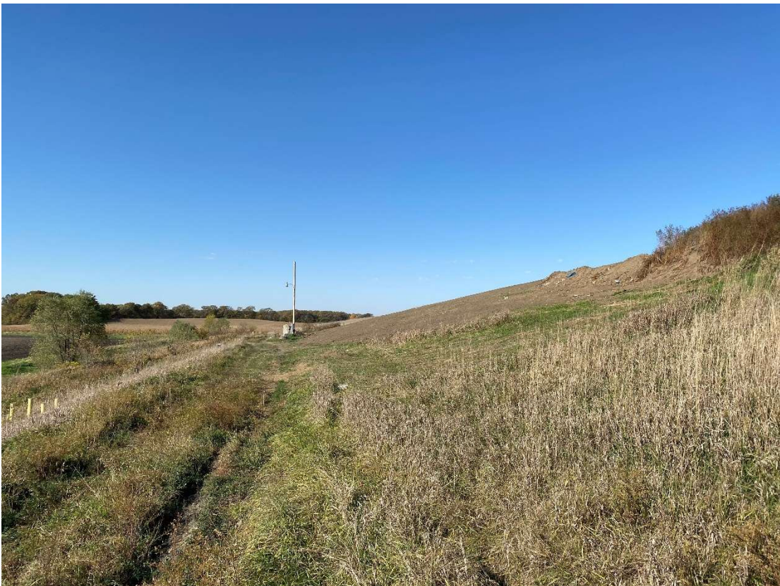
Location 7 – Looking West, Phase 2 Southern Perimeter Road and Slope
