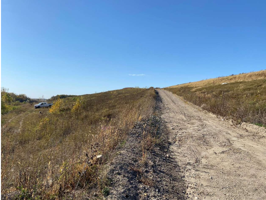
Location 10 – Looking South, Phase 2 Eastern Slope and Interior Access Road Entrance
