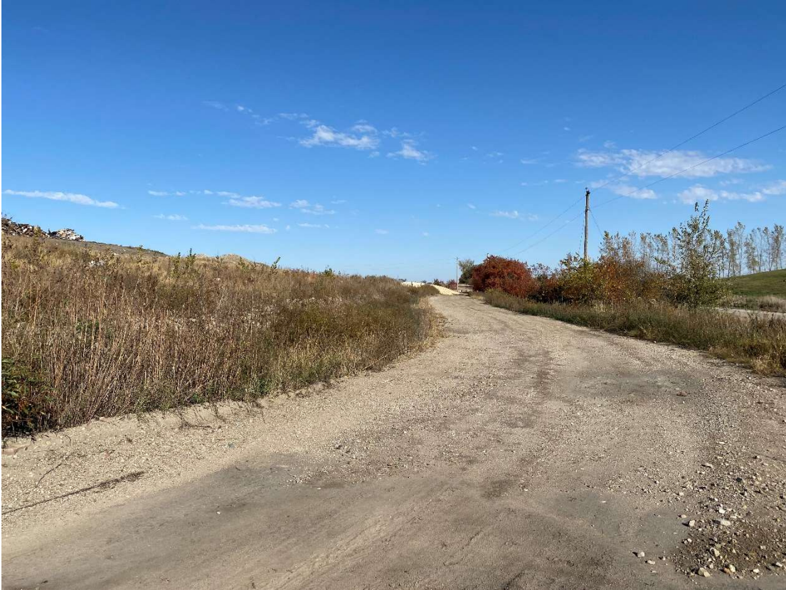
Location 9 – Looking North, Phase 2 Eastern Berm
